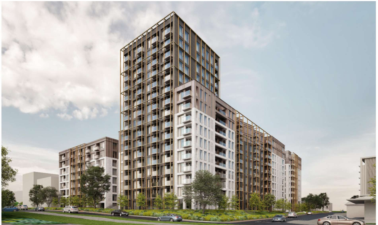
Figure 7 View of proposed development elevation onto Blackthorn Road at the corner with Carmanhall Road (Source: MDO Architects)
